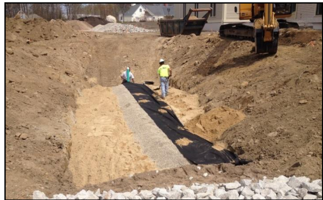
Bio-retention drainage system installation
